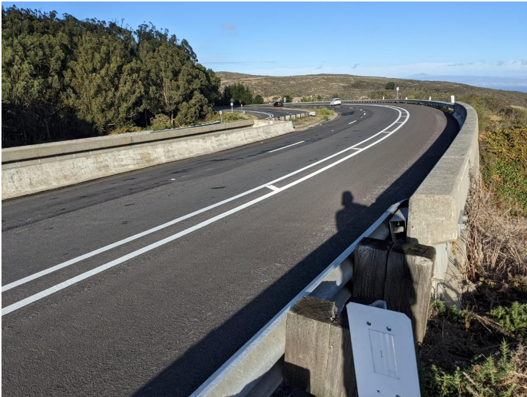
Figure 1: New Buffered Bicycle Lane and Reduced Lane Widths on Guadalupe Canyon Parkway
