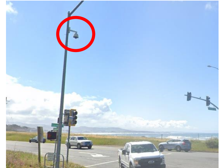
Dome Camera (Closed-circuit television)
