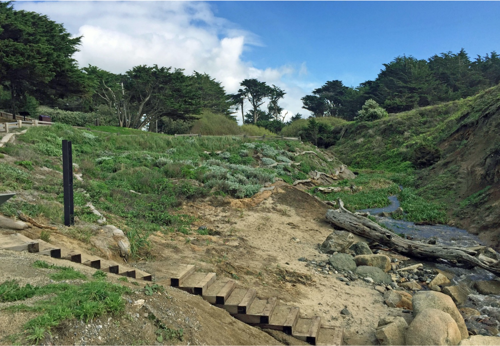
Native landscape restoration at reef access trail along San Vicente Creek 2016
