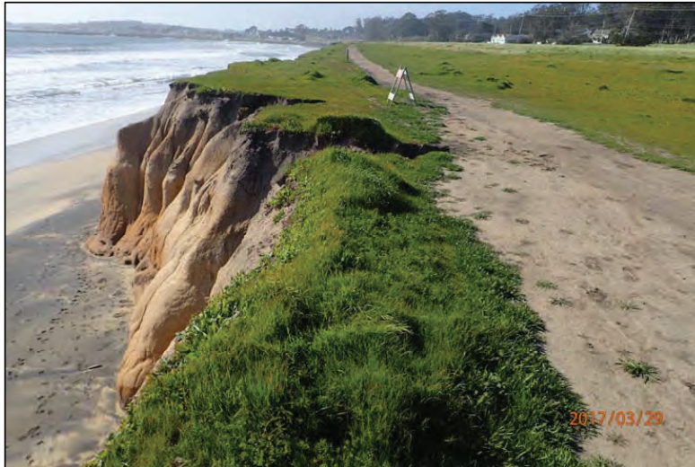
Photo 31 (Coastal Bluff Trail): View of bluff retreat looking northward along unpaved coastal trail. This photo is looking up the hydrologically connected right road reach to the gullies displayed in the previous photo.
