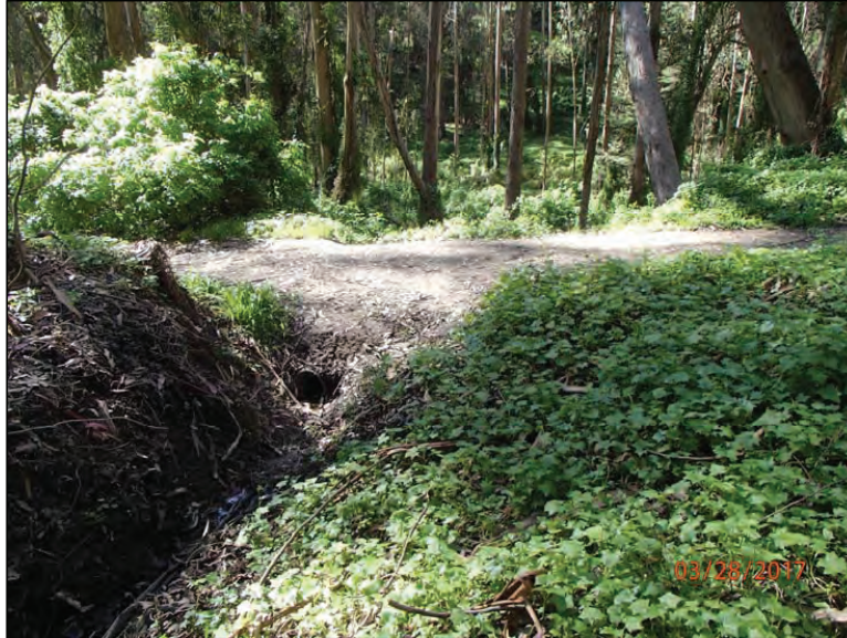
Photo 27 (Site #36): View of a culvert inlet on a small Class III stream at Site #36. This site is downstream of the pond Site #37 in the base of the quarry.
