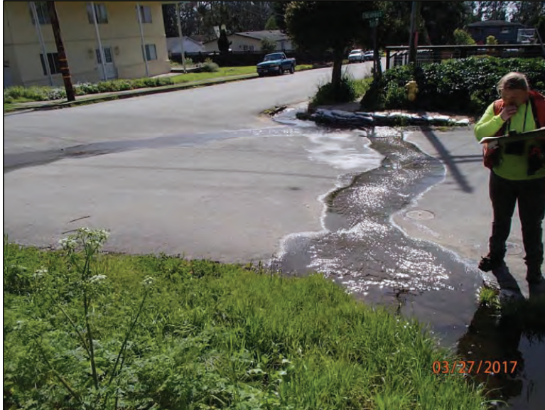
Photo 35 (Urban Drainage Interface - AOC 2): View of uncontrolled Class II stream flow exiting the Park at Santa Maria Avenue (AOC2, Map 2). Combined flow from the stream and road surface runoff travel down Santa Maria Ave. The majority of the Park's drainage area evacuates the Property into the residential area downstream at this location.
