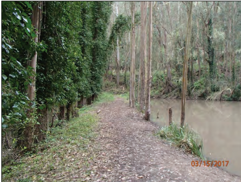
Photo 5 (Site #4): View of the levee associated with the on-stream reservoir Site #4, looking west-southwest across the top of the dam face.
