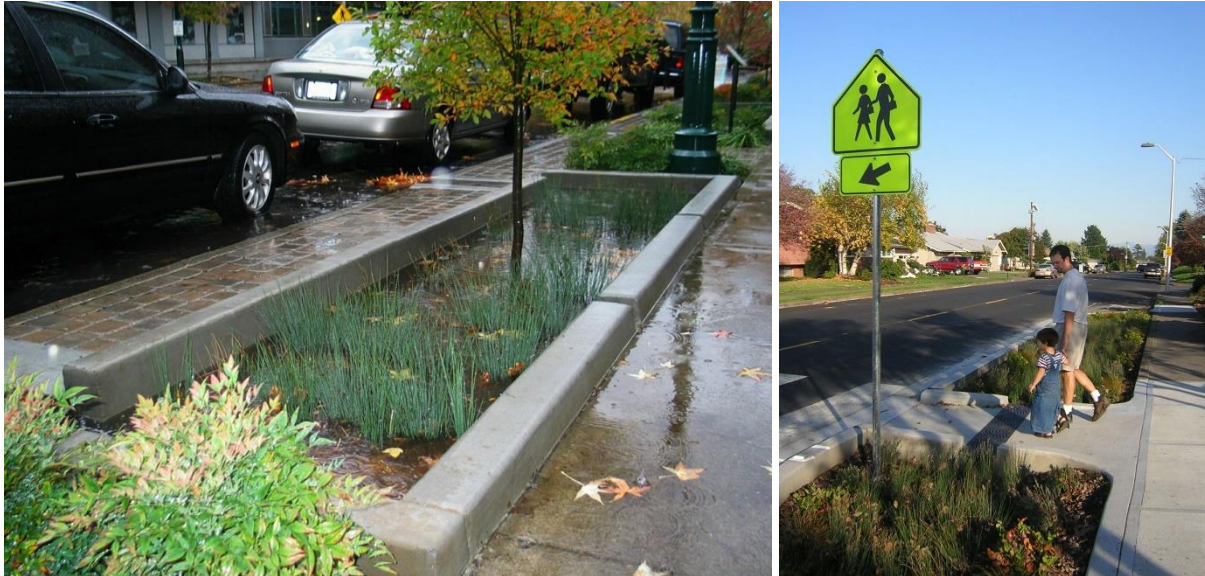
Figure 4-2. Example stormwater planter box (SMCWPPP 2009) and bioretention curb extension at a crosswalk (SMCWPPP 2009).
