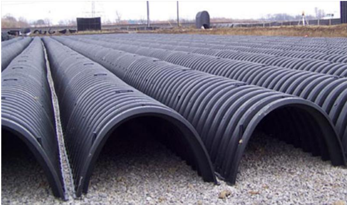
Figure 4-1. Subsurface infiltration system installation under a parking lot (SMCWPPP 2016a).
